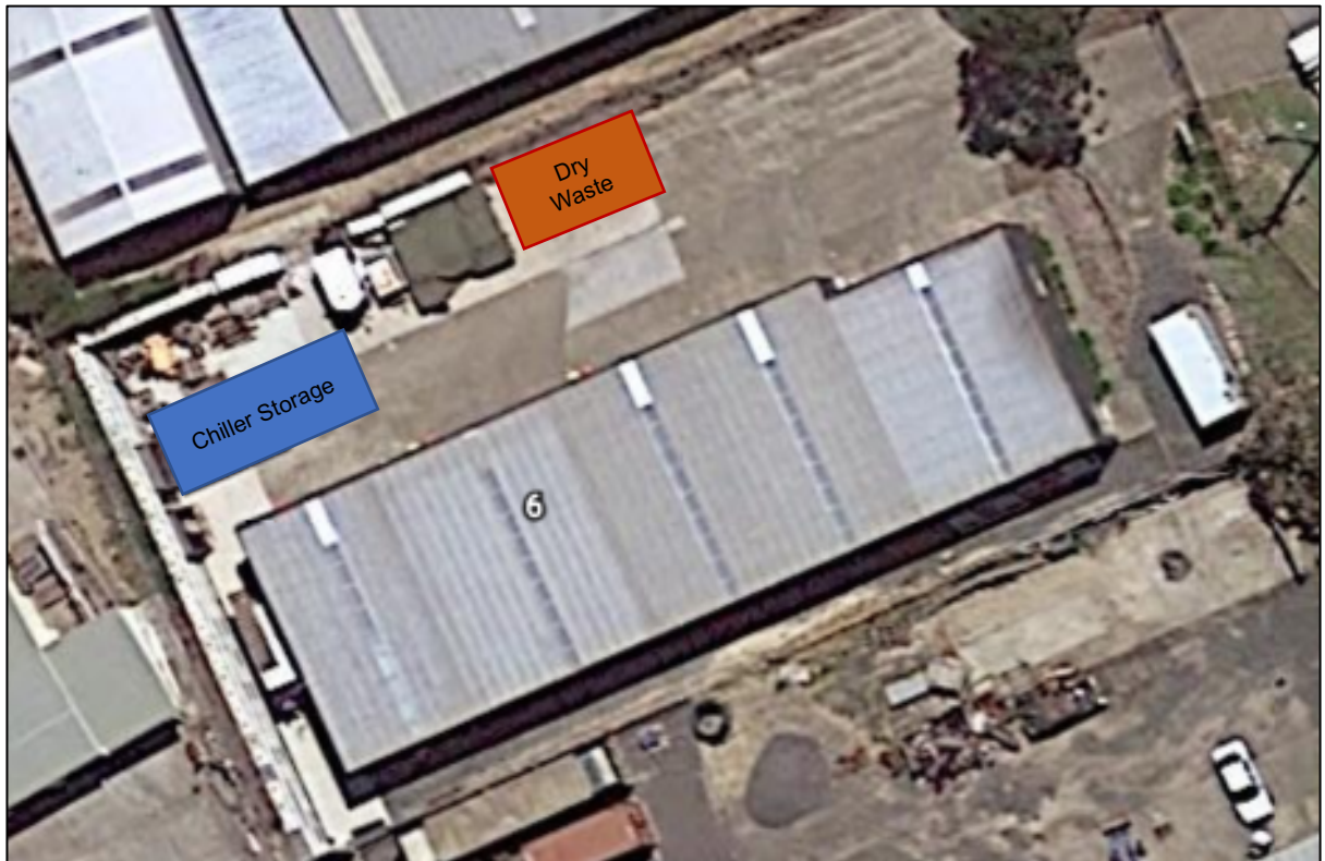
Figure 1: South Coast Mariculture Processing Facility, 6 Bolton Road Huskisson – chiller (blue) and dry waste (orange) storage areas.
